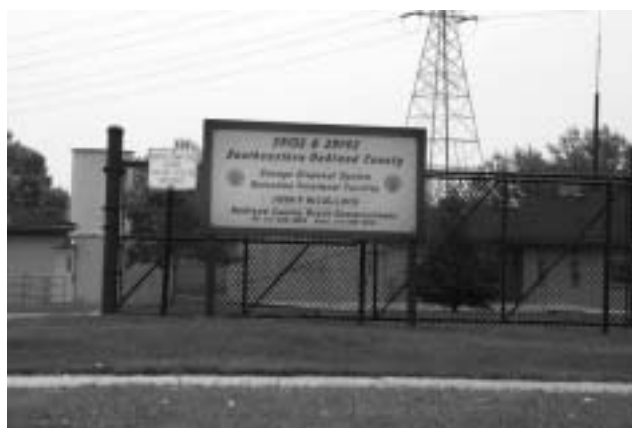
Sewage disposal facility in Madison Heights.
