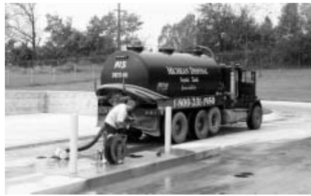
Oakland County's Septage Unloading Facility located in Pontiac provides a convenient, controlled, and cost-efficient process to dispose of septage from residential septic tanks and sediment from municipal catch basins. The facility features easy access for loading and unloading septage, diversion provisions for storm water surface runoff, and watertight construction to prevent septage leaks and groundwater infiltration.
