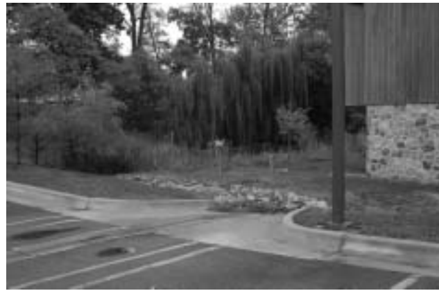
Auburn Hills is managing parking lot runoff by capturing and treating the runoff instead of directing it to the storm drain.
