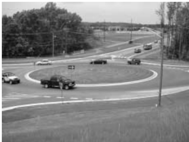
Roundabout in Rochester Hills.
